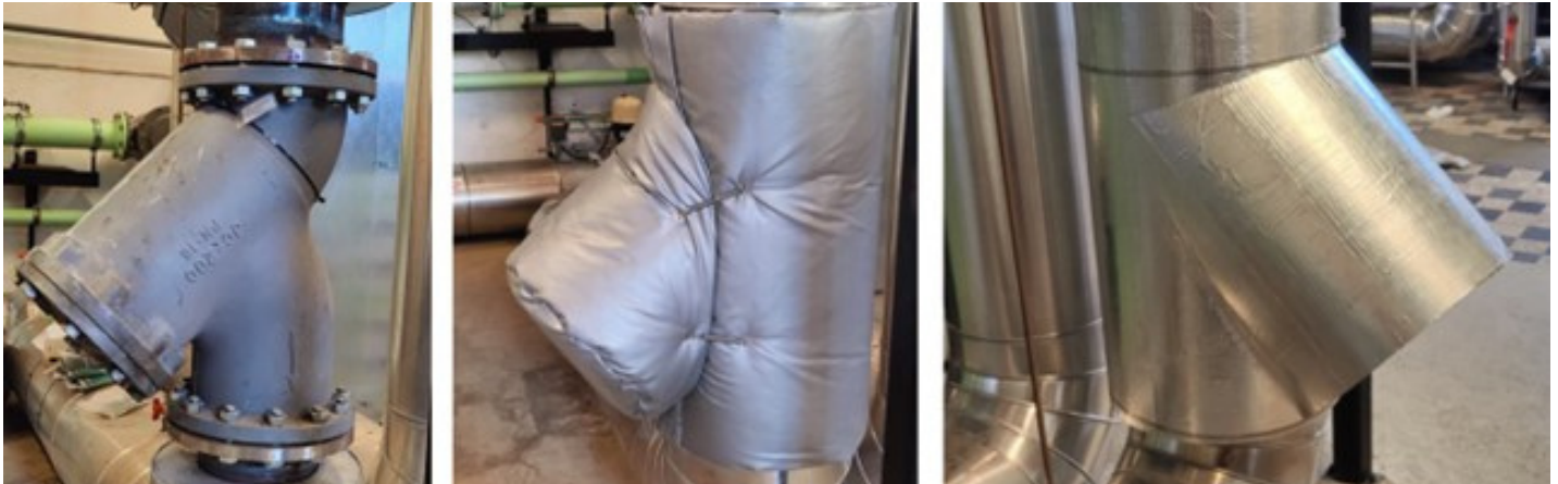
Dirt arrester installed in a district heating pump station.
