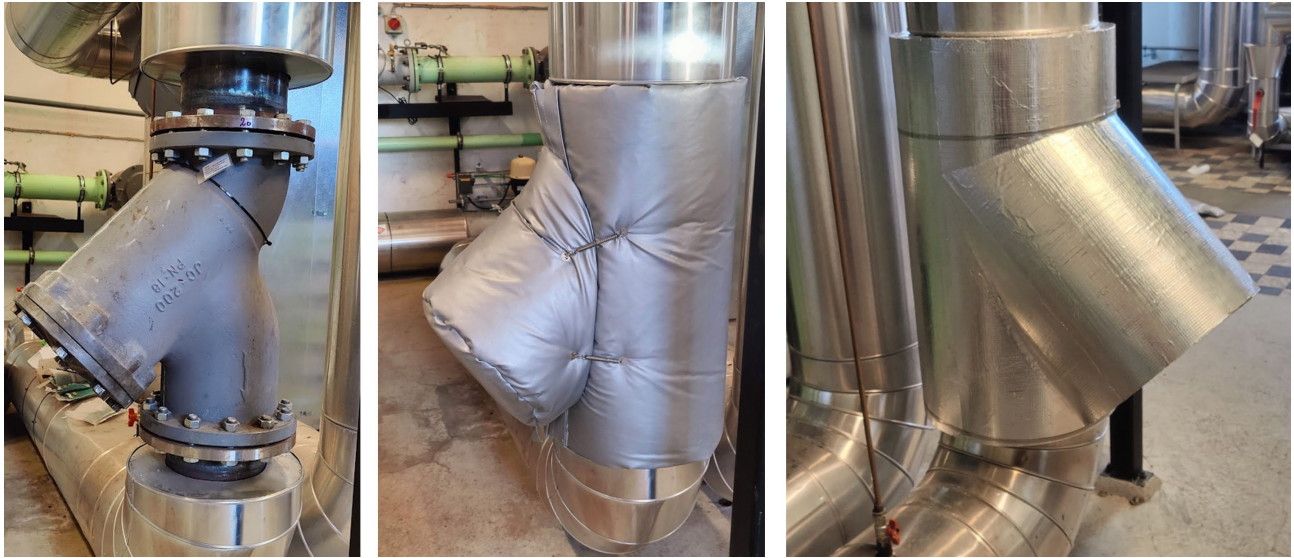
Figure 4: Dirt arrester installed in a district heating pump station.
